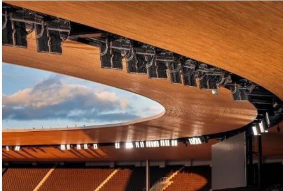
The optics made from PLEXIMID® TT50 are a significant component of the new Sirius® floodlight system as they focus the light, thereby increasing efficiency, as can be seen here in Helsinki.
